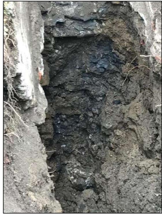
Plate 4 Mudstone at base of quay wall
