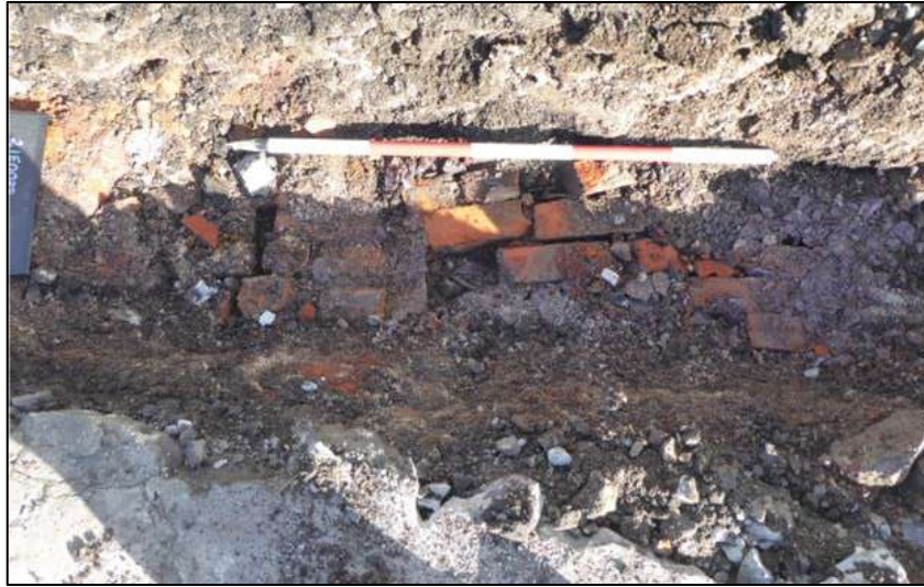
Plate 6 Unbonded red brick floor, test pit 5
