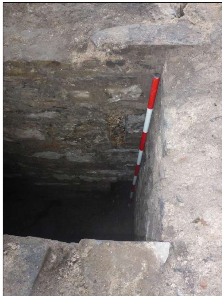
Plate 21 Test Pit 8 showing air flue at the base of the ranging rod, view to north-northwest
